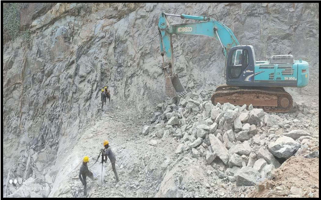
Workers with personal protective equipments
